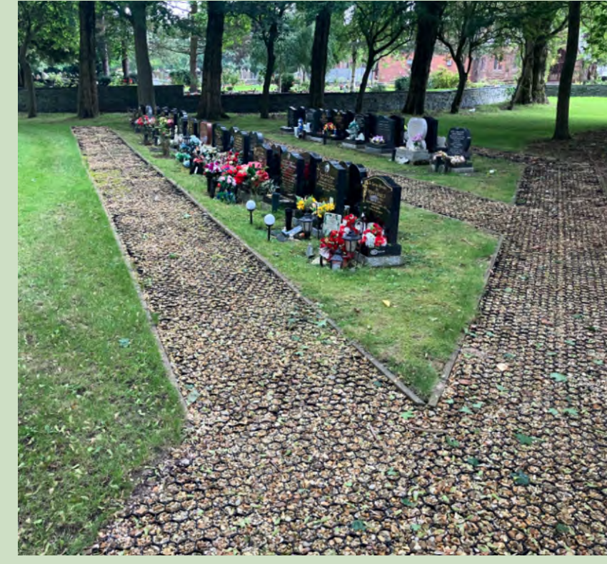
Permeable Paving to store surface water and slow runoff.
