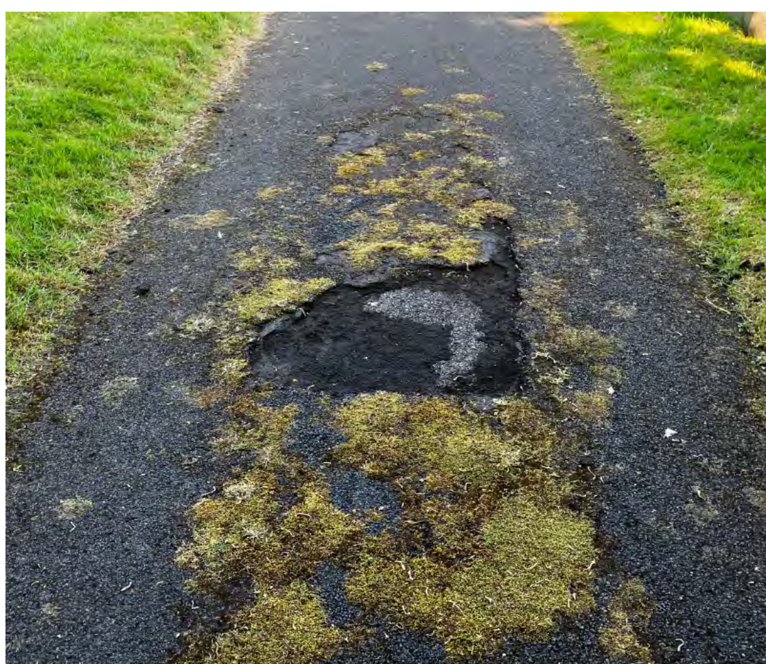
Failing old sections of pedestrian paths need to be repaired to avoid claims so rationalisation of path surfacing and hardstanding will reduce this ongoing burden.
